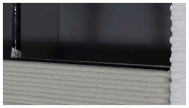
3-D printing builds things by layering material via a computer-programmed robotic arm.
